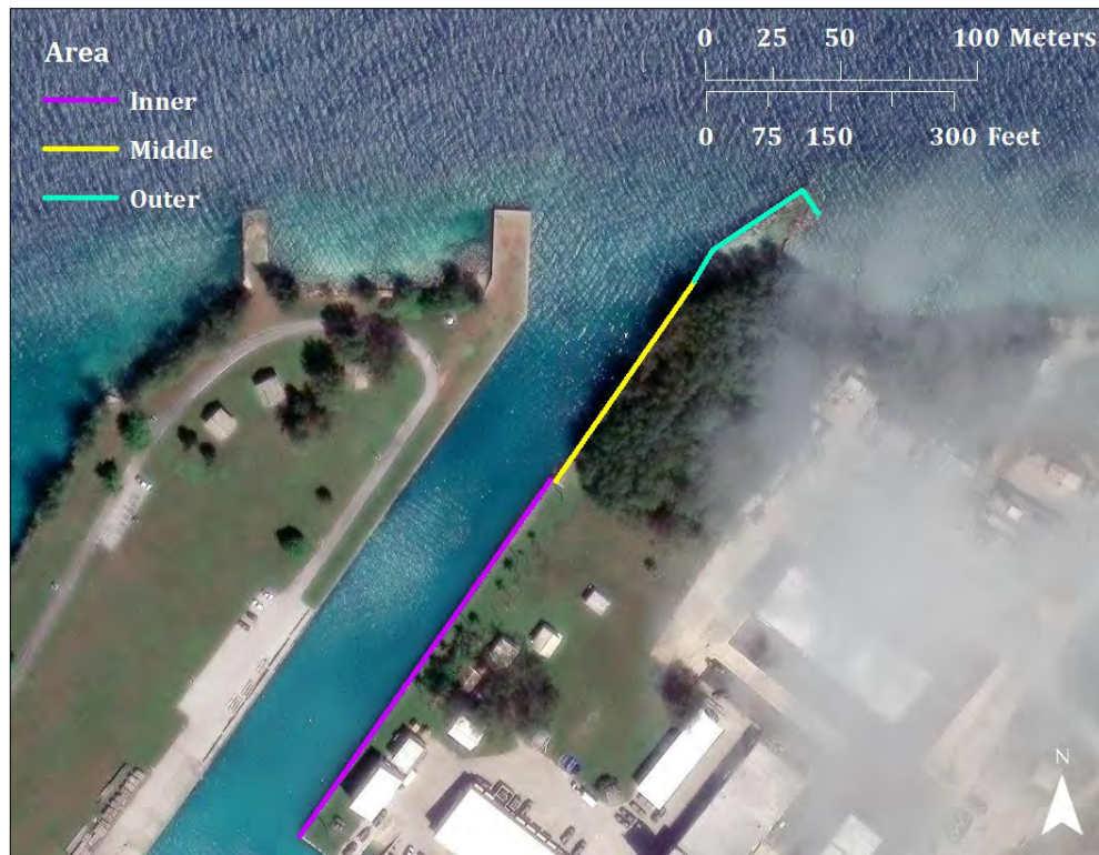
Figure 11. Representation of EOD seawall areas: 1) Outer, in teal; 2) Middle, in yellow; 3) Inner, in purple.
